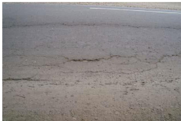
Gambar 2. 5 Cekungan ( Bumb and Sags )
