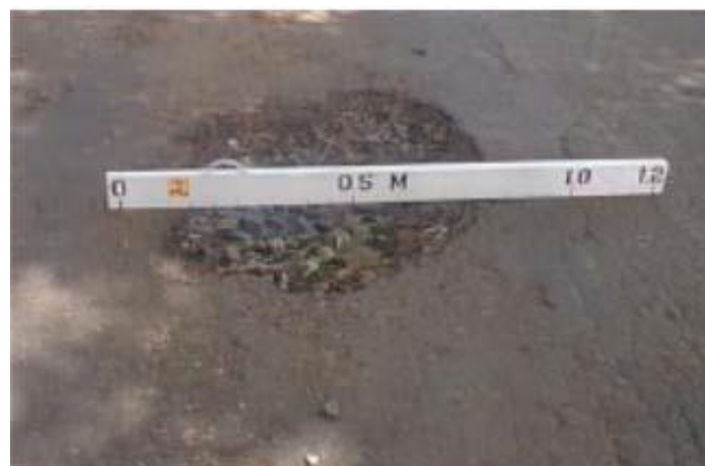
Gambar 2. 14 Lubang ( Pothole )
