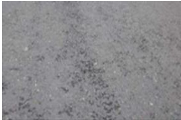
Gambar 2. 20 Pelepasan Butir (Weathering/Raveling)
