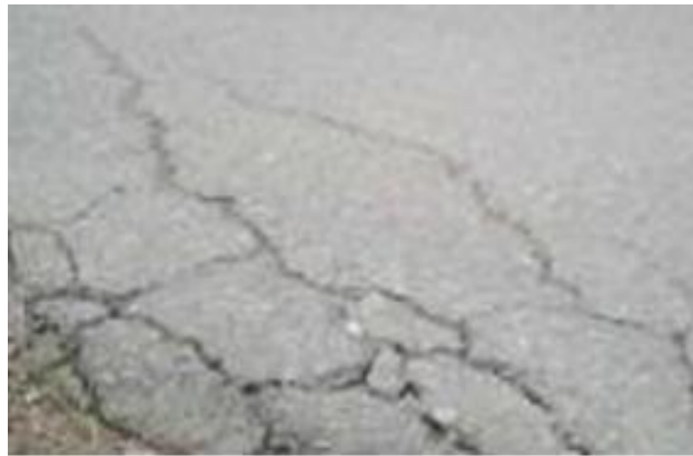
Gambar 2. 8 Retak Samping Jalan (Edge Cracking)
