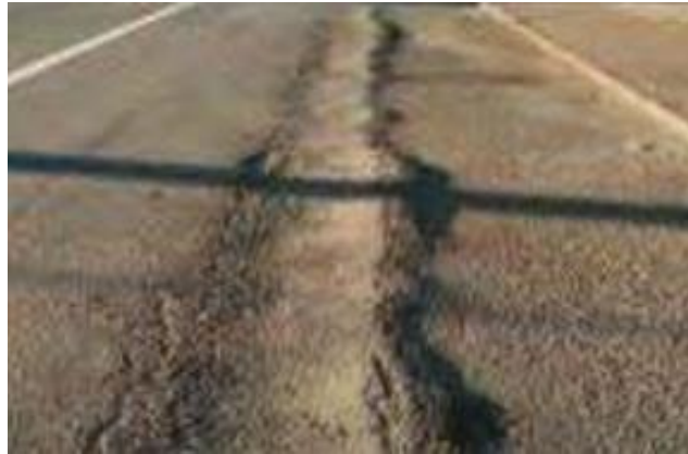
Gambar 2. 16 Alur ( Rutting )
