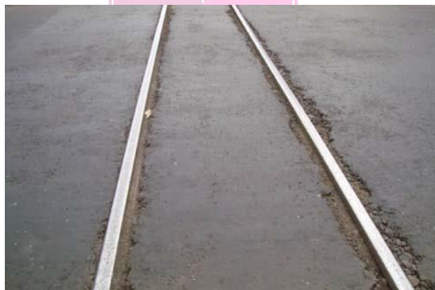
Gambar 2. 15 Rusak Perpotongan Rel ( Railroad Crossing )
