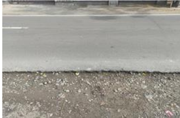
Gambar 2. 10 Penurunan Bahu Jalan (Lane/Shoulder Drop Off)
