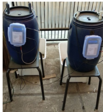
2: Installation of an irrigation tank monitoring system
